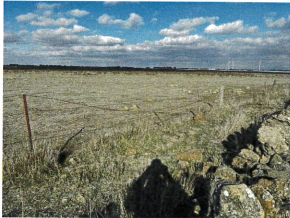
Photo 2: Fencing with loose wiring
